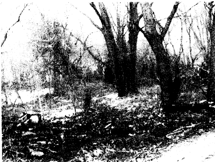
After Clearing of Brush and Saplings - View from South Street Looking North February 22, 2007
