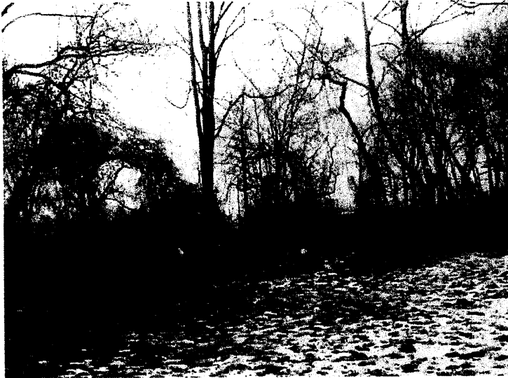
After Clearing of Brush and Saplings - View from Center Street Looking Northeast February 22, 2007
