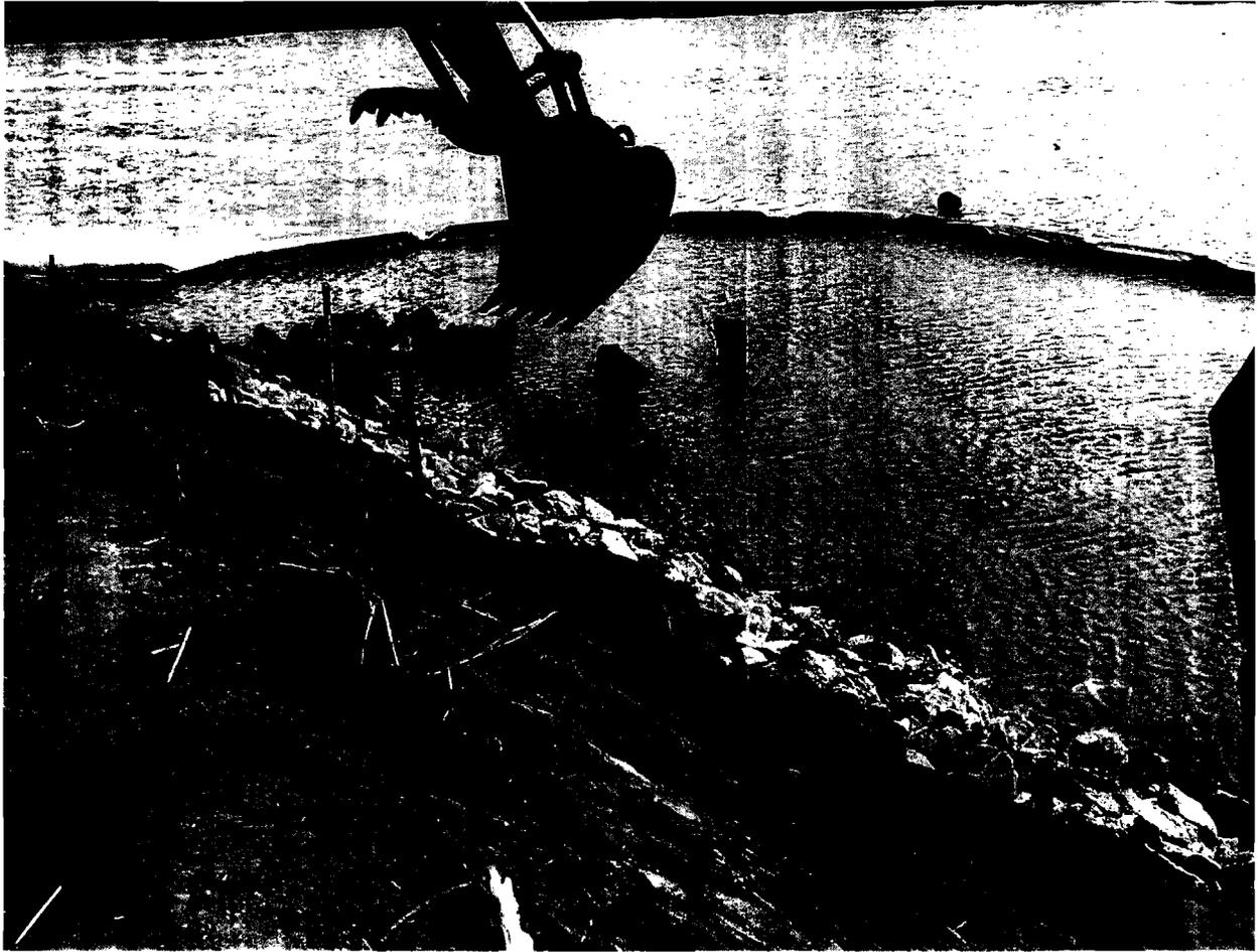
*Figure 6. Erosion control/bank stabilization under construction along the perimeter of the active portion of the plant, March, 2008. Similar measures are proposed to be employed for OUI.*
